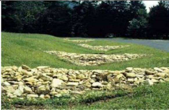
a check dam made of stone
